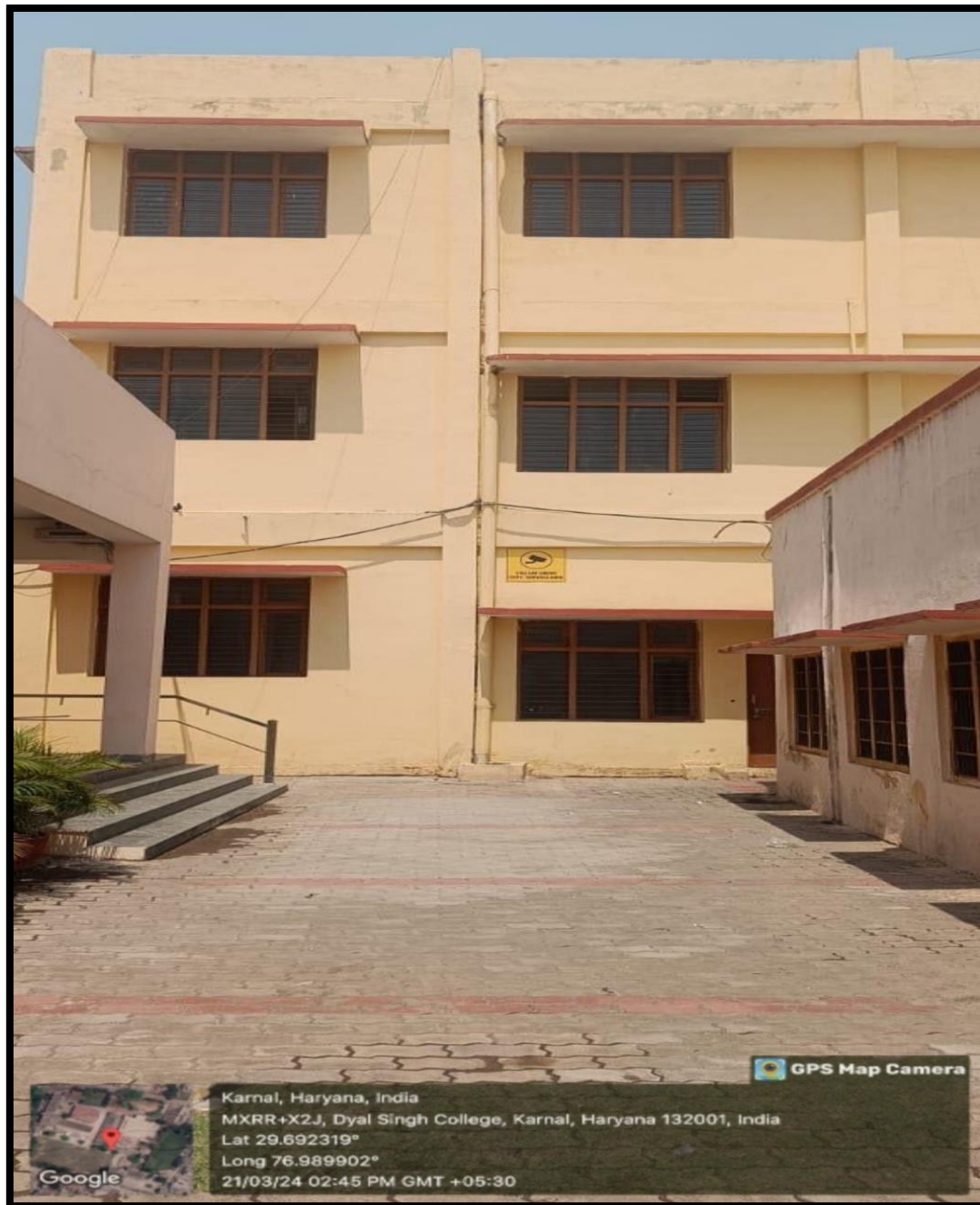
Rain water Harvesting System
